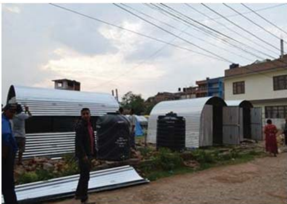
Assembling mobile houses
